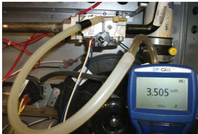
FIGURE 30 - MANOMETER MEASURING GAS MANIFOLD PRESSURE
