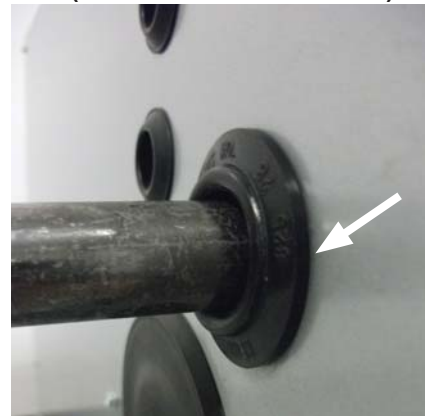
FIGURE 27 - FURNACE GAS PIPE CONNECTIONS (NOTE RUBBER GROMMET)
